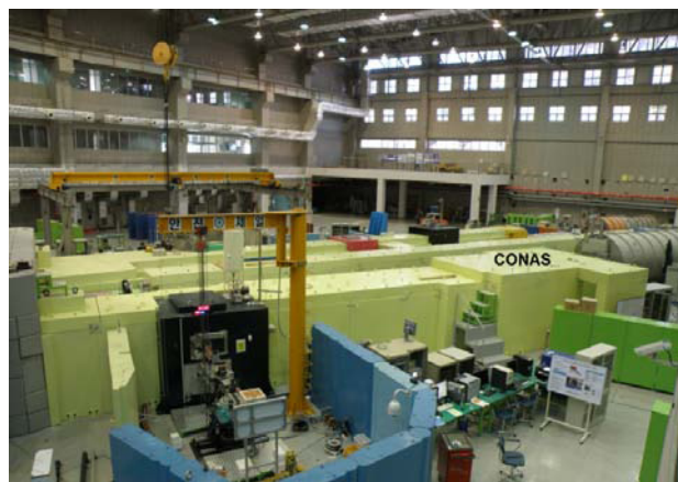
Figure 2. Cold Neutron Activation Station, where a cold neutron PGAA (CN-PGAA) was installed.
